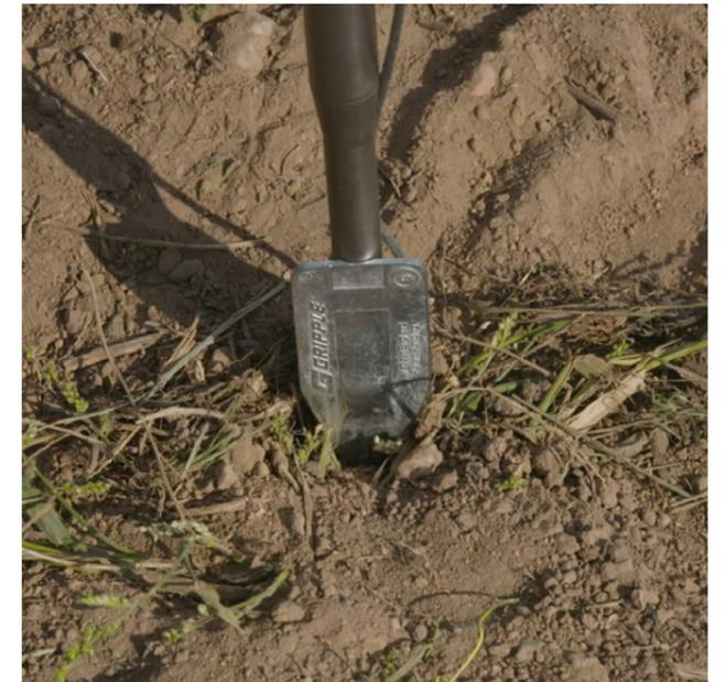
APEX anchor being driven into the ground.
